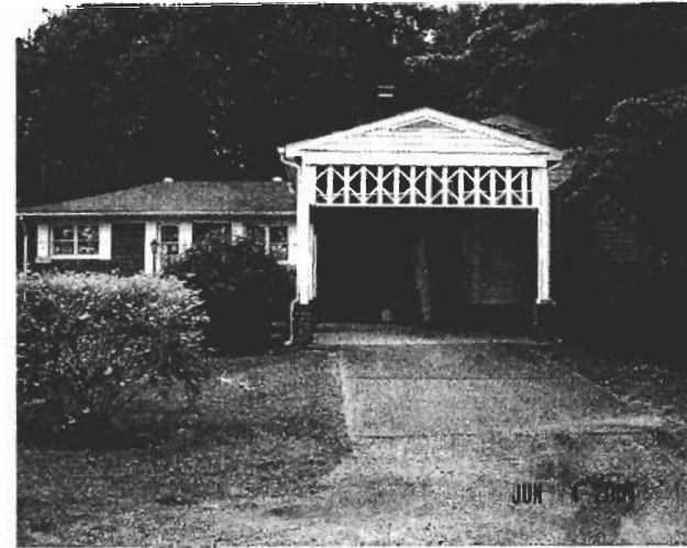
Right: Driveway for the private residence to which the Playhouse is attached.
