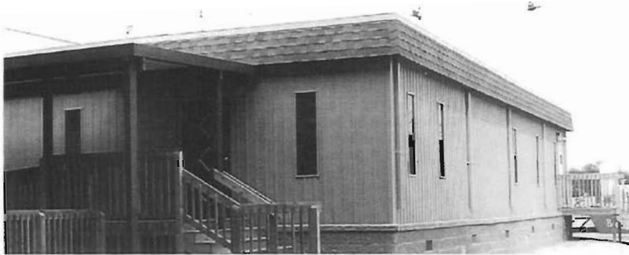
Similar Example of Proposed New Modular Building. Siding and roofing materials will match the existing main church building
