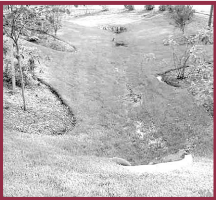
Stormwater management can be incorporated into landscaping to create an aesthetically pleasing stormwater detention basin, as seen on Jamestown Road.
