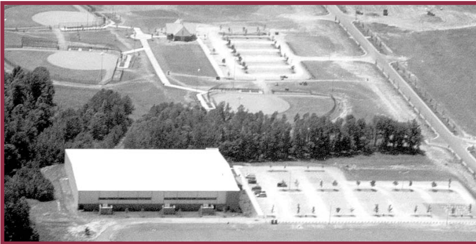
Phase II of the District Park Sports Complex , part of the Parks and Recreation Master Plan, was completed by adding two concession/restroom facilities, lighting and utility installations
