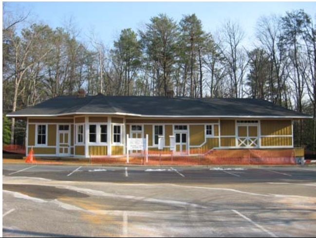
Front Elevation View, Depot Phase II Exterior Restoration complete.
